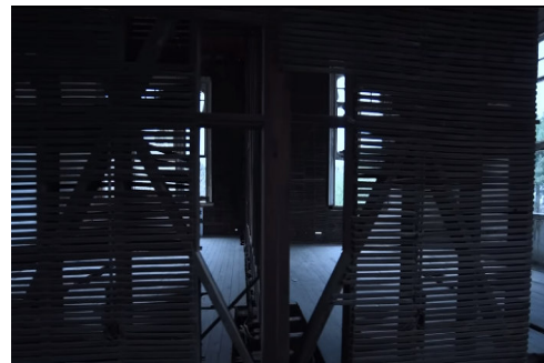
Fig. 16. Bağdadi covered interior walls of the timber frame system (İbrahim Akgün)
