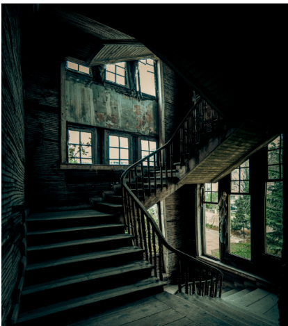
Fig. 6. The interior of the stair tower (İbrahim Akgün)
