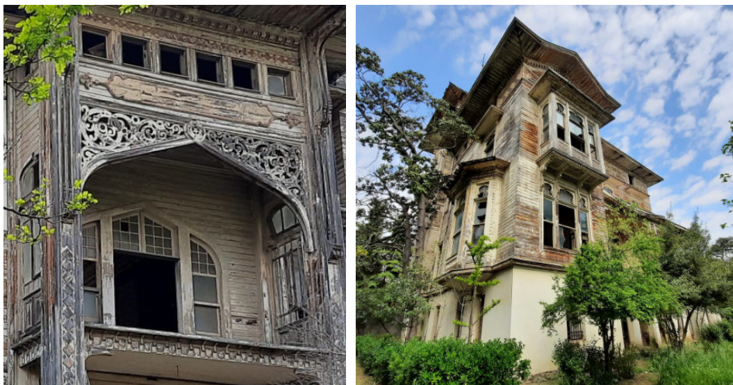
Fig. 11. Above: The oriel window of the room overlooking the sea on the upper floor and the supporting wooden buttresses called fūruş (Author). Below: The wooden Seljuk/Art Nouveau pointed arch in front of the upper floor sofa (Author)
