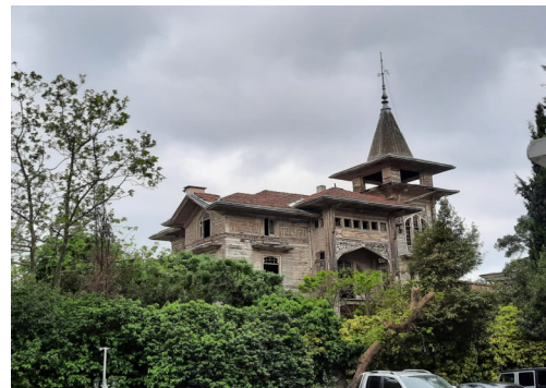
Fig. 7. The observation balcony of the cihannüma , which is crowned with a conical, pyramidal cone that overlooks the top of the stairwell tower at a higher elevation than the building itself (Author)
