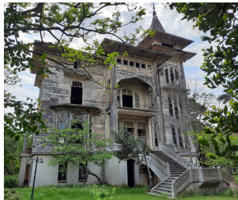
Fig. 5. The wide-eaved triangular room projecting on the left side of the sofa (parlor) (Author)
