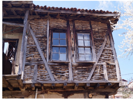
Fig. 10. Basketweave-filled timber framework system. Detail. Şile Akçakese Village (Author)
