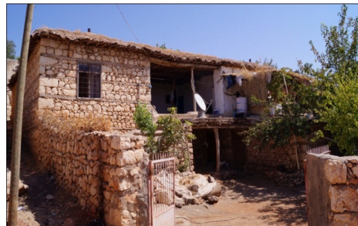
Fig. 14. Use of a wooden beam on a stone wall (Author)
