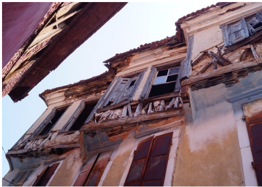
Fig. 6. Stone infilled timber-frame system. Kula (Author)
