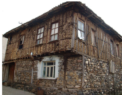
Fig. 4. The timber frame brick infilled system. Bursa, Derekızık Village (Author)
