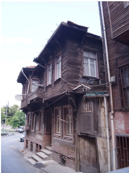
Fig. 18. Ribbed Wood Sheathing used in a timber framework system, Istanbul (Author)
