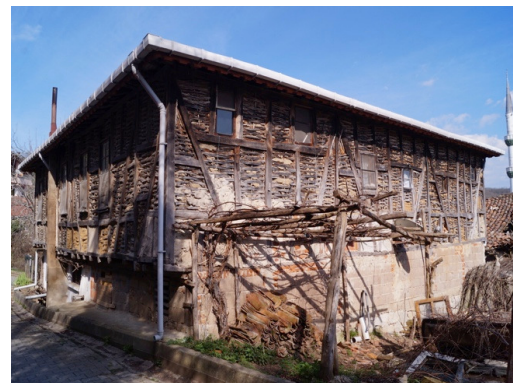
Fig. 11. Basketweave-filled timber framework system. Şile Akçakese Village (Author)
