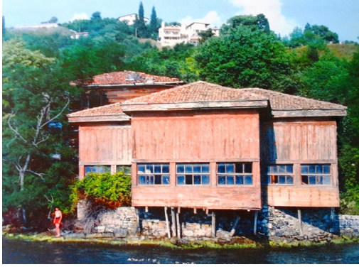
Fig. 20. An example of vertical wood sheathing on timber framework. Köprülü Amcazade Hüseyin Paşa Waterside Mansion [18]
