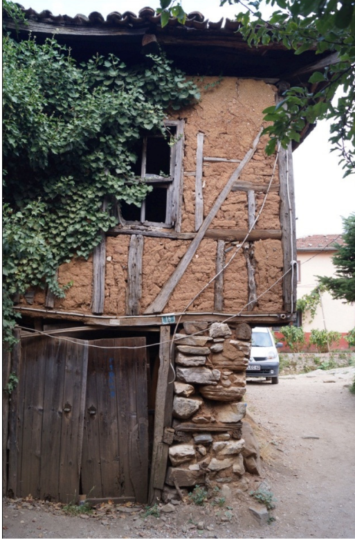
Fig. 5. Mudbrick-filled ( kerpiç ) timber frame system. Cumalıkızık (Author)
