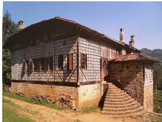
Fig. 7. Cell-filled/stuffed wall system [6]
