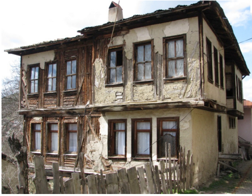
Fig. 9. Dizeme infilling in the timber framework ( çatki ) system. Mudurnu (Cultural Portal, Mudurnu Bolu)
