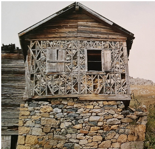
Fig. 8. Houses built in the muska or triangular amulet system [6]
