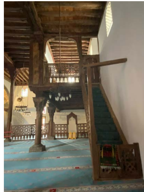
Fig. 15. Wooden balustrades of Sultan's mahfil (Author)
