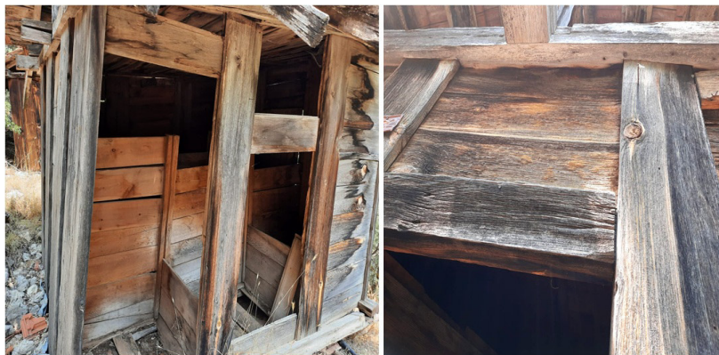
Fig. 11. Right: The head beam of the top wall construction is fitted into the posts in the “kurt boğazi” joint system (Author). Left: Channels ( kiniş/keniş ) opened in the posts and the timber planks fitted into the channels ( kiniş/keniş ) (Author)
