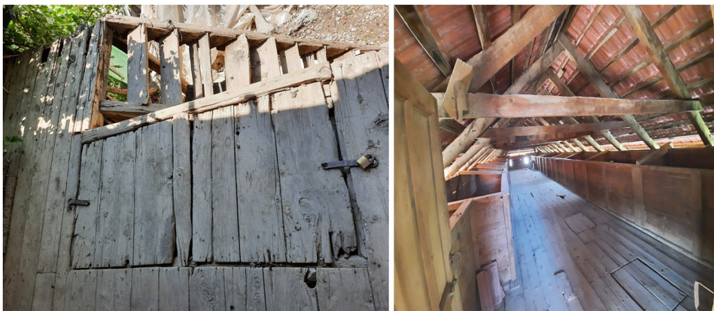
Fig. 16. Right: Interior of Elmalı “ Ağa/bey ” granaries. Gübse with wooden lids on the base of the granary (Author). Left: Granary lids on the base of the “ Köşk ” (Author)
