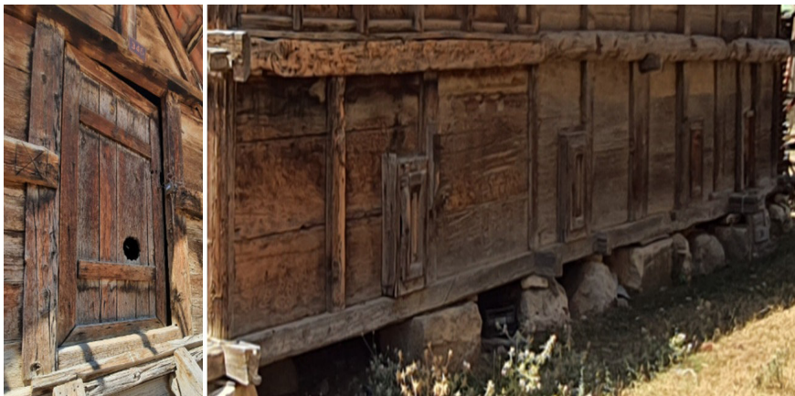
Fig. 7. Right: The side facades of the “ aga/bey ” granaries in Elmalı have unloading lids called “ çeşme ” (fountain) (Author). Left: The “ cat holes ” (locally kedilik ) on the granary doors in the Elmalı area (Author)
