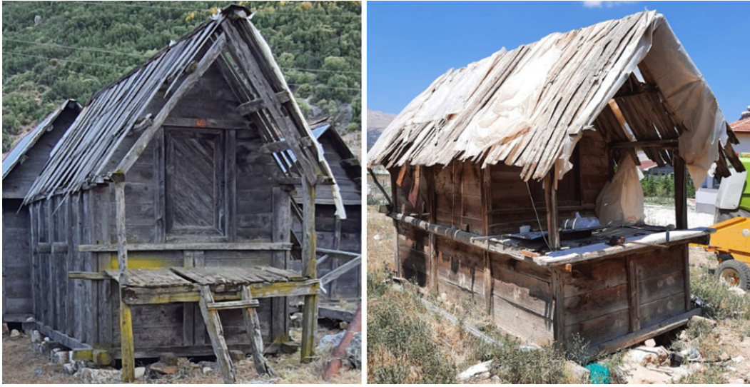
Fig. 18. Padavra type of roof (Author)
