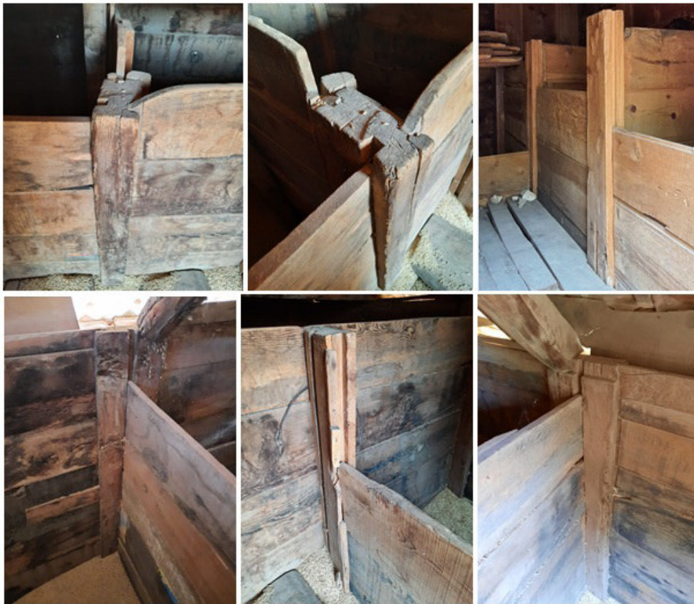
Fig. 17. Göz/gübse in the sections of the granary, built in the “çalma boğaz” joint system. Channels ( kiniş/keniş ) opened in two and three directions (Author)
