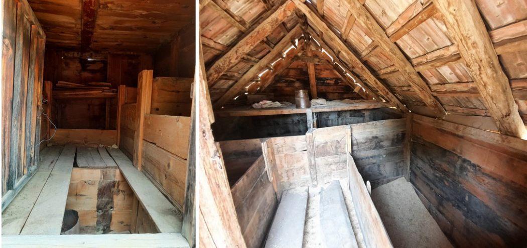
Fig. 15. Compartments ( gübse ) below the granary floor, on the side, and in the back (Author)
