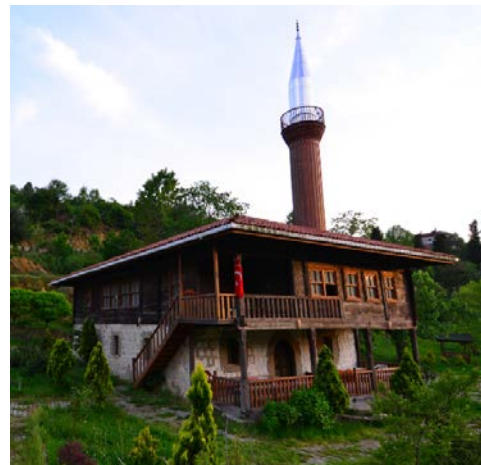
Fig. 6. A mosque built in the kurtboğazı interlocking technique. Rize Hemşin Mosque (Sinan Doğan)
