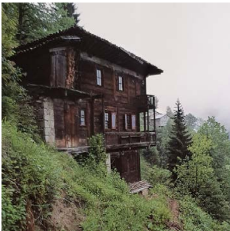
Fig. 5. Examples of mosques built in the kurtboğazı interlocking technique. Right: Rize Çamlıhemşin Şenköy (Omokta) Mosque [6]
