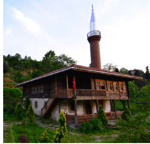
Fig. 6. A mosque built in the kurtboğazi interlocking technique. Rize Hemşin Mosque (Sinan Doğan)
