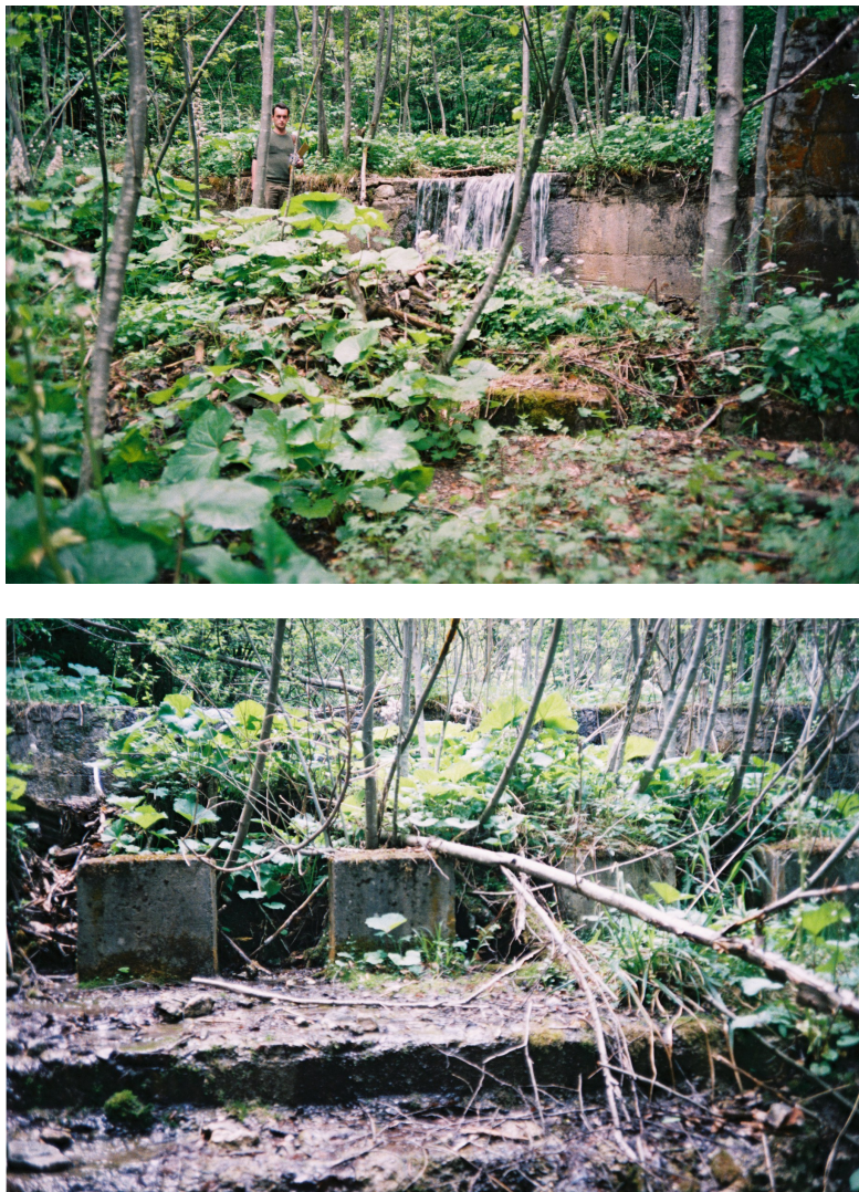
Fig. 1. Examples of uncontrolled installation of forest vegetation on the managed torrential network in the Upper Târlung Watershed. Photo: Clinciu, 2003
