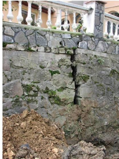
Fig. 3. *The large opening of the settlement joint*
