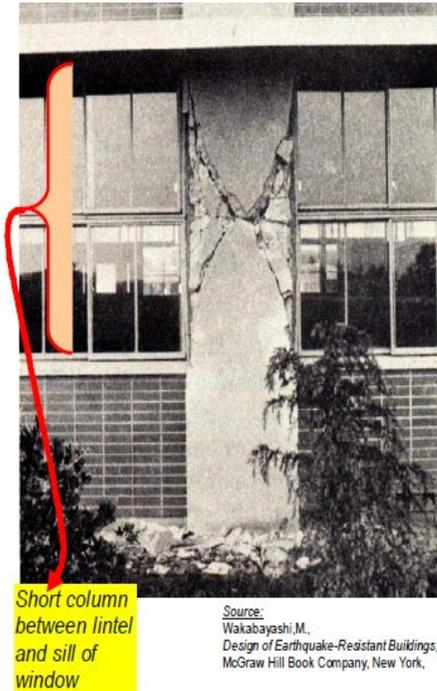
Fig. 5. *Short columns damaged, in the form of X-shaped cracking [2]*
