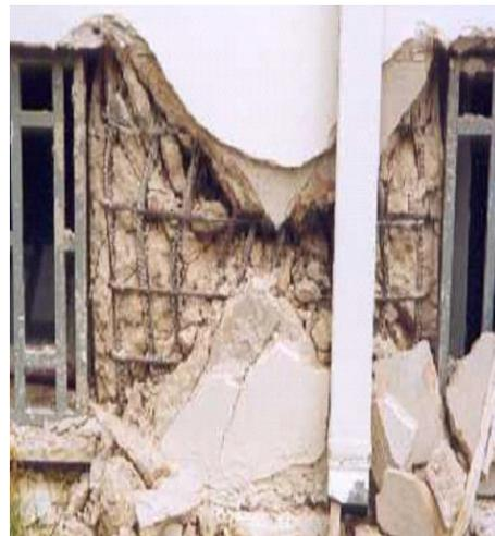
Fig. 6. *Short columns damaged, in the form of X-shaped cracking*
