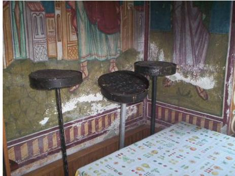
Fig. 4. *Degraded frescos, due to ascending humidity*
