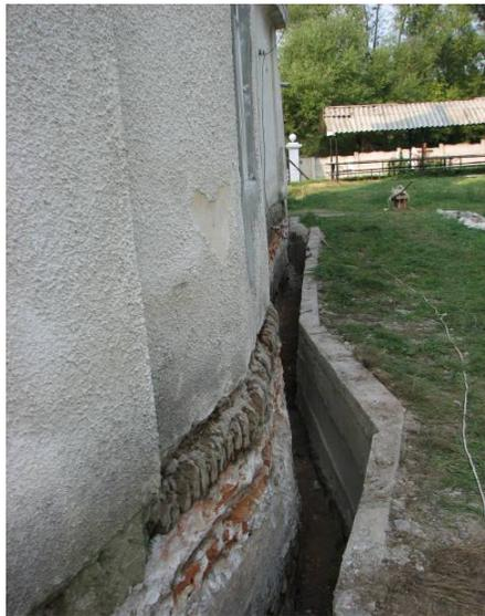
Fig. 12. *Preparing foundation wall for the intervention from outside the church*
