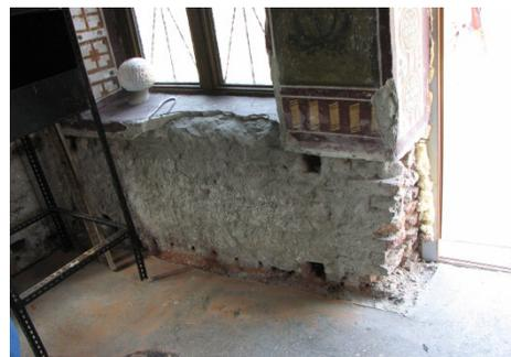
Fig. 10. *Continuous belt of holes at the bottom of brick wall*
