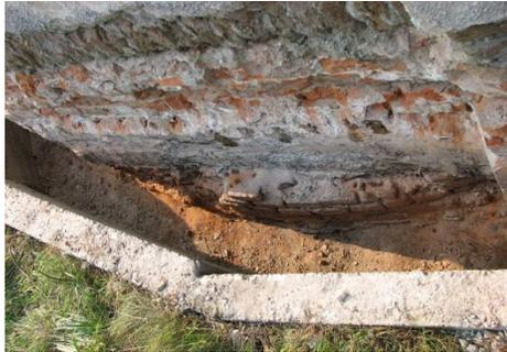
Fig. 11. *Intervention at the exterior side of the wall*
