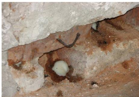
Fig. 9. *DryZone gel inserted in holes made at the bottom of brick wall*
