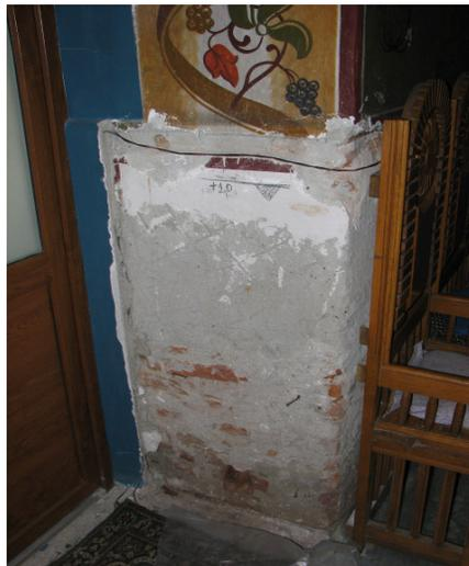
Fig. 8. *Setting the right elevation before making holes in brick wall*
