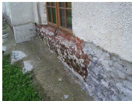
Fig. 3. Degraded wall, due to capillary moisture
