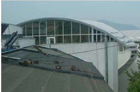
Fig. 2. Photo of the “Solar House”
