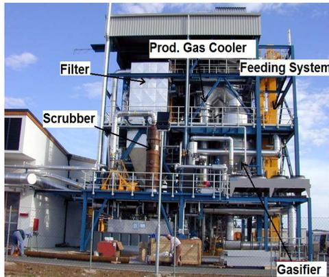
Fig. 4. View over the CHP Güssing [6]
