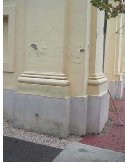
Fig. 4. Variation of capillary moisture in wall height
