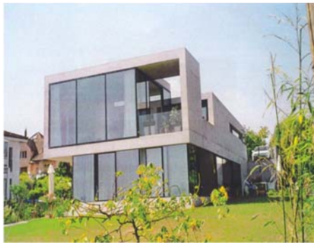
Fig. 3. Single-family house with VIP-Multiplac wall elements
