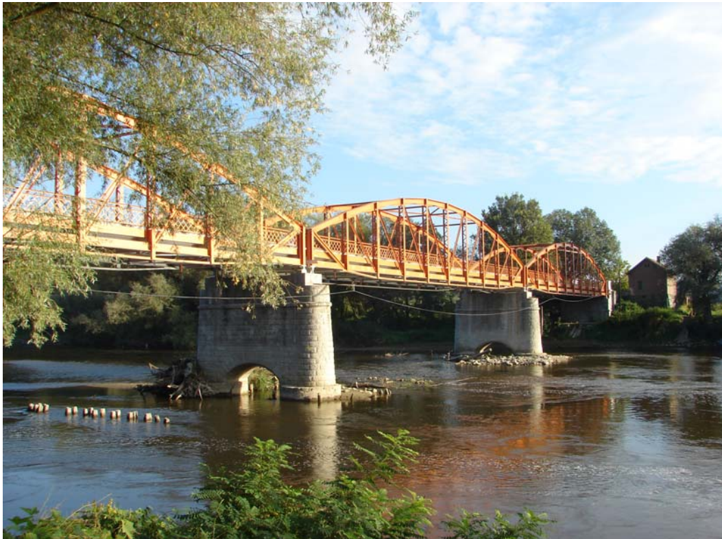
Fig.12 Savarsin Bridge after rehabilitation
