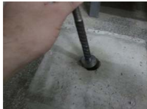
Fig. 2. Installation of the head connector into the \Phi 30mm damp hole.
