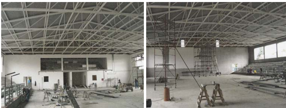
Fig. 1. Photos of the sports hall prior to testing under trial loads
