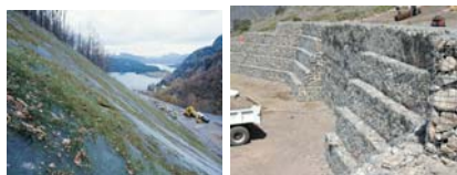
Fig. 3. Prevention of soil erosion and landslides
