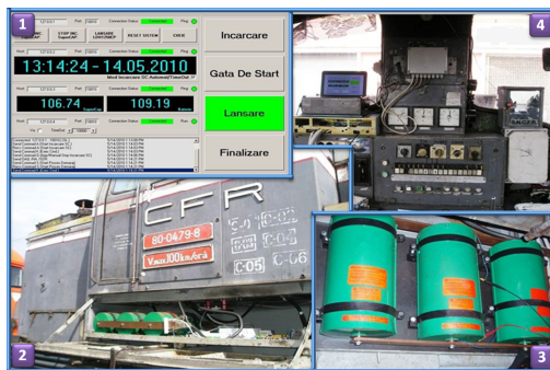
Fig. 2. The starting system prototype implemented on LDH1250HP [11]:
