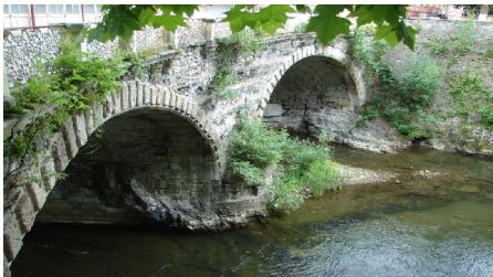
Fig. 11. The bridge infrastructure
