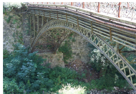
Fig. 2. The main resistance structure
