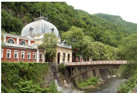
Fig. 1. The “Iron Bridge”
