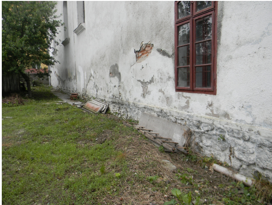
Fig. 2. Variation of capillary moisture in wall height
