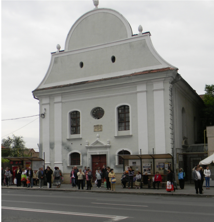
Fig. 4. Capillary moisture at the main façade wall
