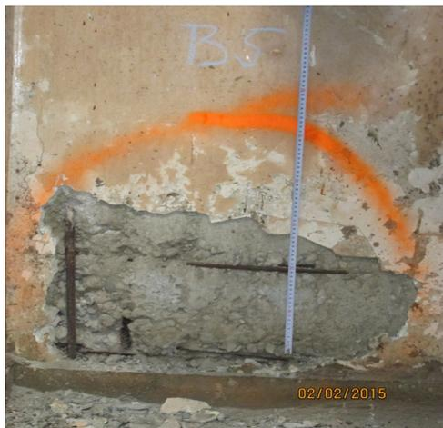
Fig. 5. *Highlight the degradation through concrete carbonation – B5 pillar in B axis*
