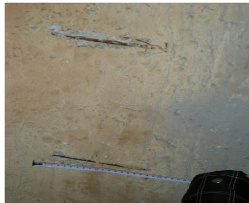
Fig. 3. *Highlight the insufficient cover concrete layer – A7 pillar in A axis*
