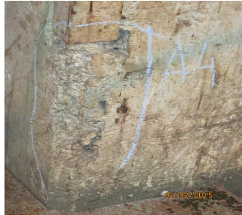
Fig. 2. *Highlight the indents and concrete segregation – A4 pillar in A axis*
