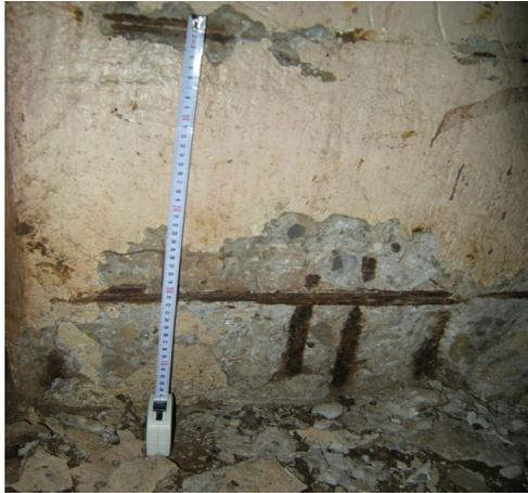
Fig. 4. *Highlight the degradation through concrete carbonation; reinforcement corrosion – A2 pillar in A axis*
