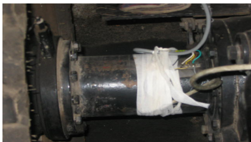
Fig. 5. Mounting the capture signal wires from sensors
