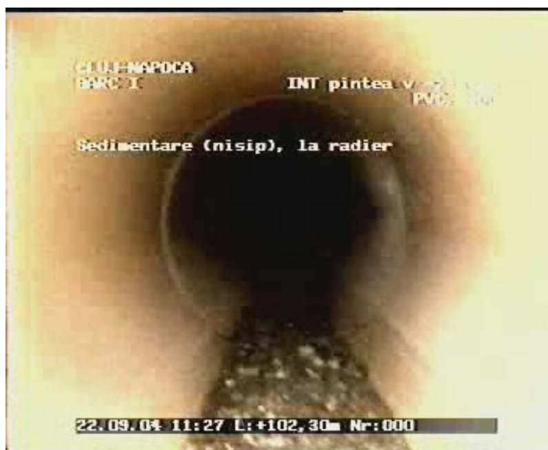
Fig. 2. Small deposit of sediments (below 10%). The sewer section capability of transporting used water is not yet affected significantly. The picture illustrates the second category of faults.
