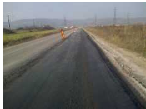
Fig. 11. Protection of the recycled layer with a cationic emulsion layer
