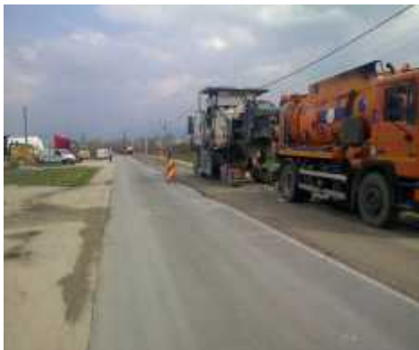
Fig. 8. Cold recycling in site: mixing equipment and water tank
