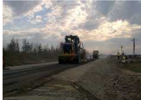
Fig. 9. Layers disposal with the auto grader
