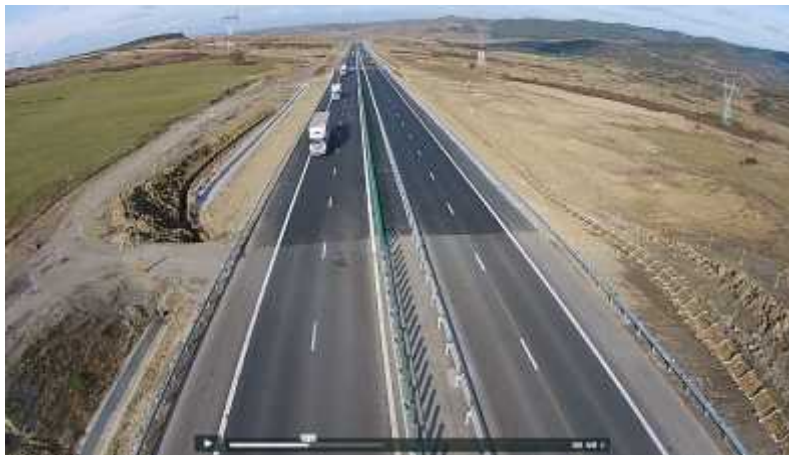
Fig. 8. Current state of works
