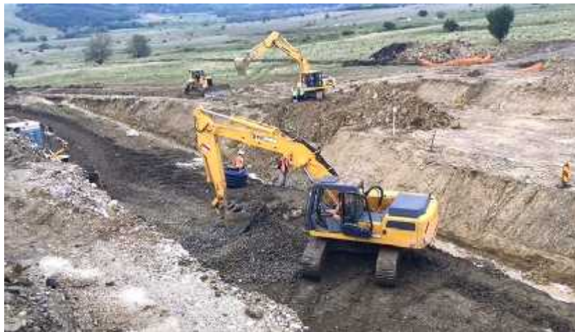
Fig. 2. Excavation of the cross drains [2]
