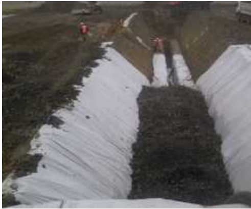
Fig. 5. Geotextil putting in work [3]
