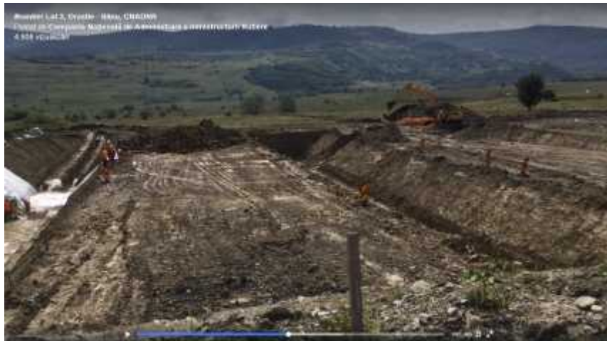
Fig. 4. Digging drain
