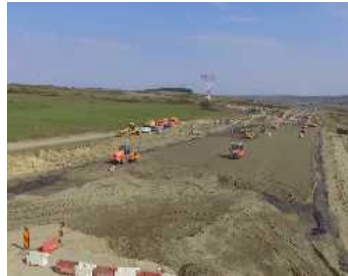
Fig. 6. Building of the embankment [3]
