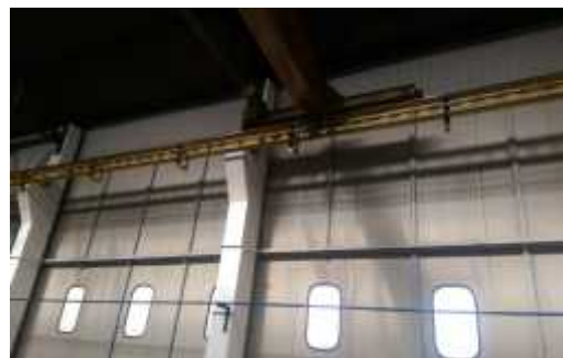
Fig. 1. Inside of existing warehouse
