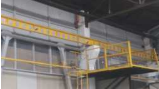
Fig. 2. Inside of existing warehouse
