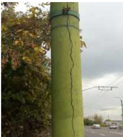
Fig. 3. Random cracks
