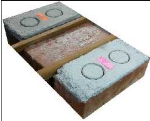
Fig. 2. Preparing the brick for plastering
