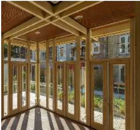
Fig. 4. Front doors and windows made of acetylated wood
