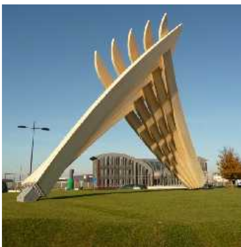
Fig. 7. Acetylated wood in architectural constructions
