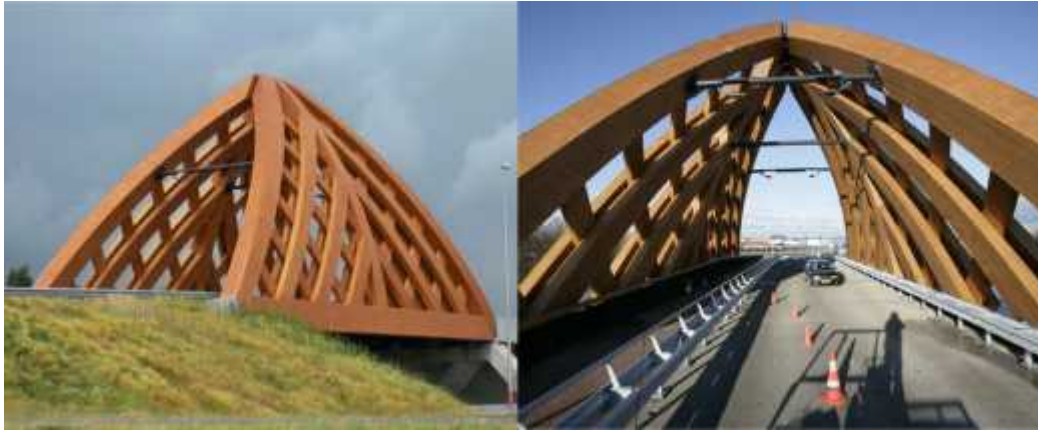
Fig. 6. Sneek Bridge in the Netherlands
