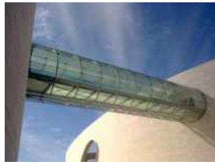
Fig. 1. *Pedestrian bridge Champlimaud Foundation in Lisbon, Portugal, a glass-steel composite structure (sbp GmbH)*
