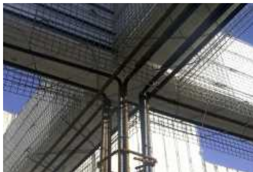
Fig. 2. Structural elements: beams
