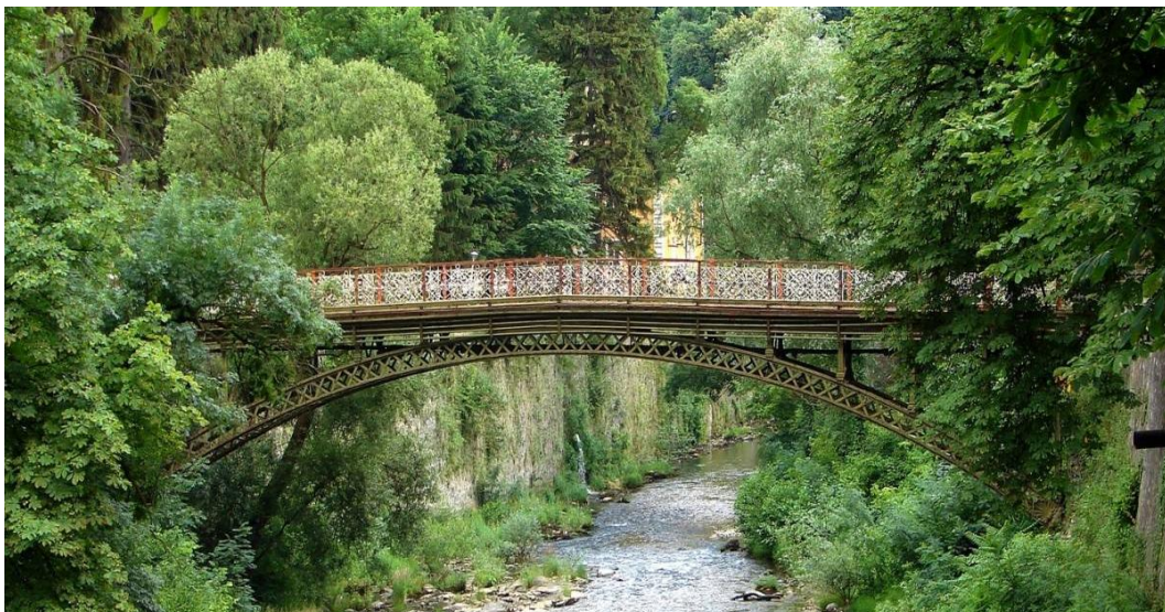
Fig. 1 General view of the arch bridge [5].
