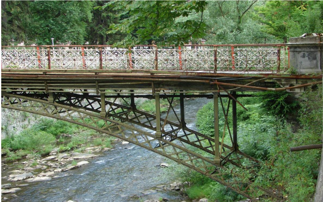
Fig. 2 Structure elements: arches, wind bracings, verticals (with ornaments) [5].
