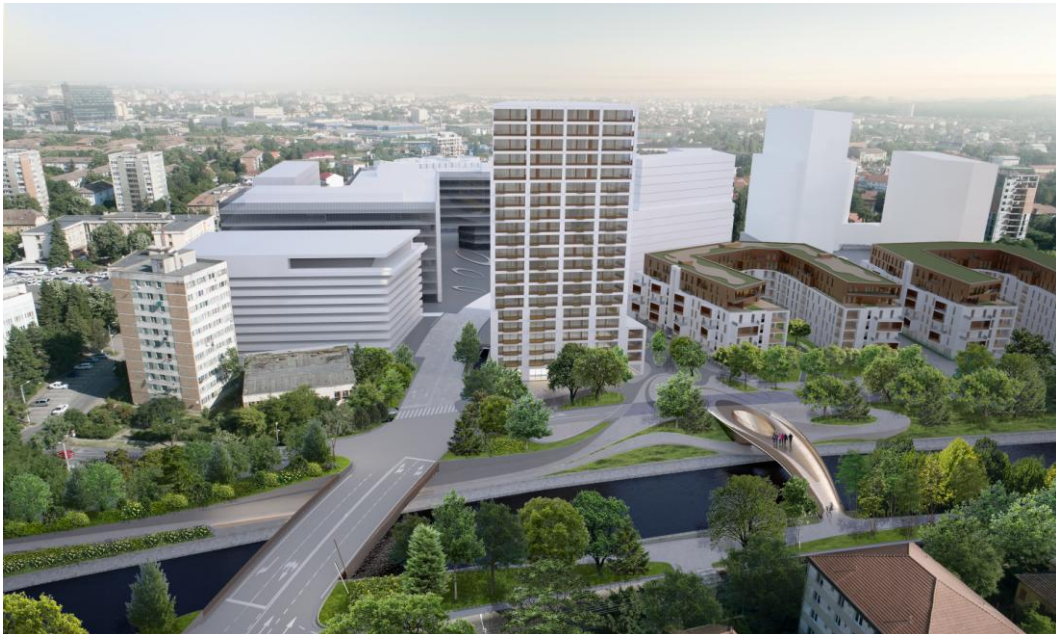
Fig. 8 The general top view of the new pedestrian bridge together with the road bridge and the surrounding new design urban area
