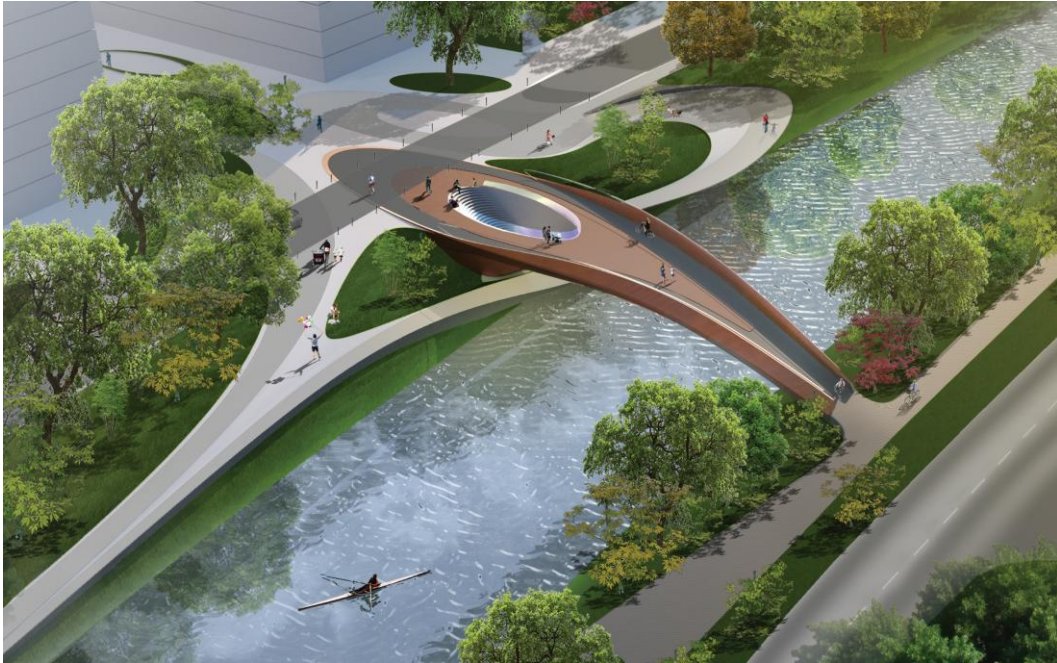
Fig. 6 General of the new pedestrian bridge [8]
