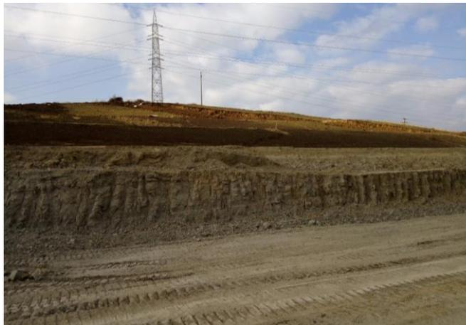
Fig. 1. *Landslide due to Loss of Stability*
