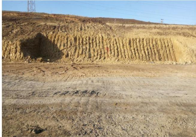
Fig. 4. The sliding plane line
