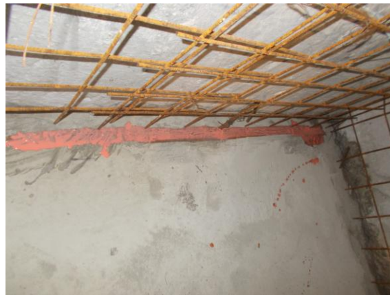
Fig. 4. Penebar primer waterstop application
