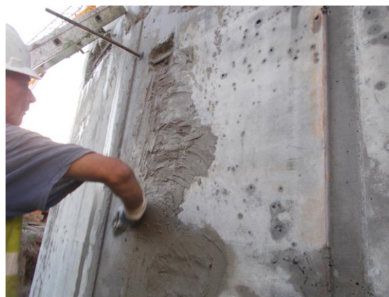
Fig. 5. Filling cracks with Penecrete mortar
