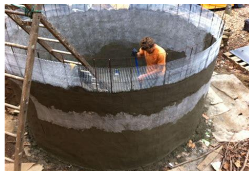
Fig. 3. Water tank under construction
