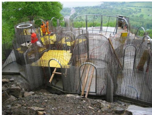
Fig. 2. House under construction
