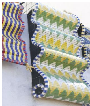
Fig. 14. Surface of corrugated closing
