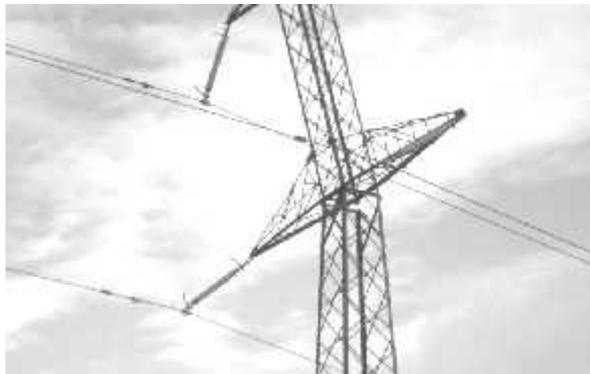
Fig. 1. *LEA type lattice steel column – bracing element failure*
