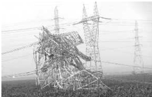
Fig. 2. *LEA type lattice steel column – collapse following the storm*
