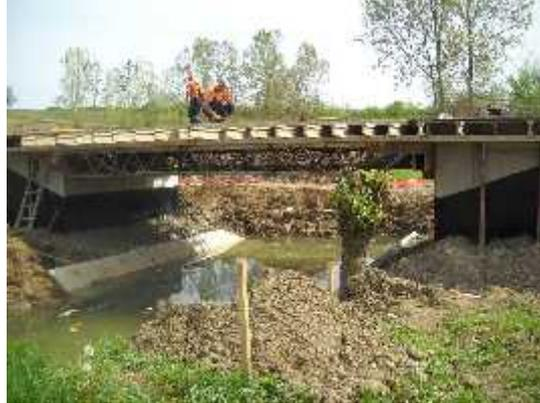
Fig. 10. *Bridge slab formwork*
