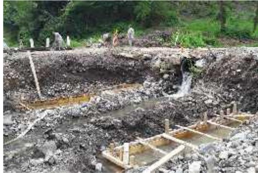
Fig. 7. *Bridge foundations*
