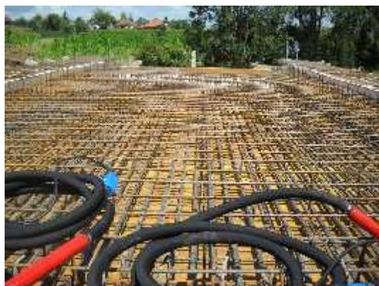
Fig. 12. *Slab reinforcement before concreting*
