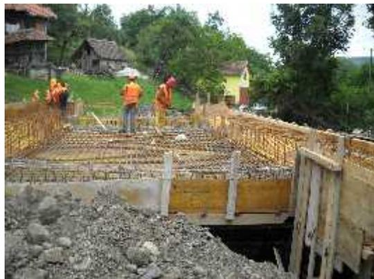
Fig. 11. *Slab reinforcement*
