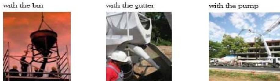
Fig. 3. Casting methods
