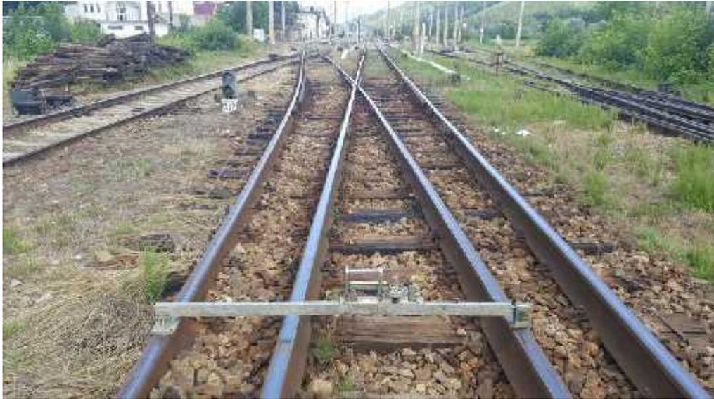
Fig. 1. *Railway switch – crossing nose*
