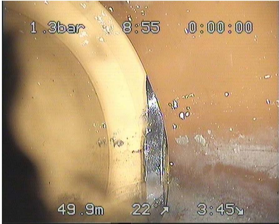
Fig. 4. Gasket expulsion at the joint due incorrect jointing technique [2]
