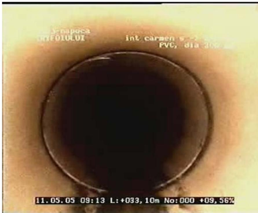
Fig. 3. *Cross-sectional deformation (ovalization) due to external overloads [2]*
