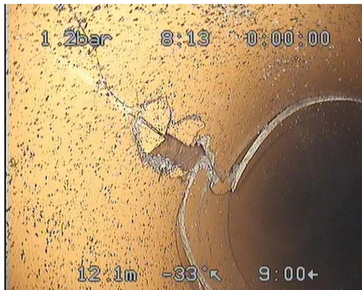
Fig. 2. Multiple cracks in the pipe wall and a portion of it is missing [2]
