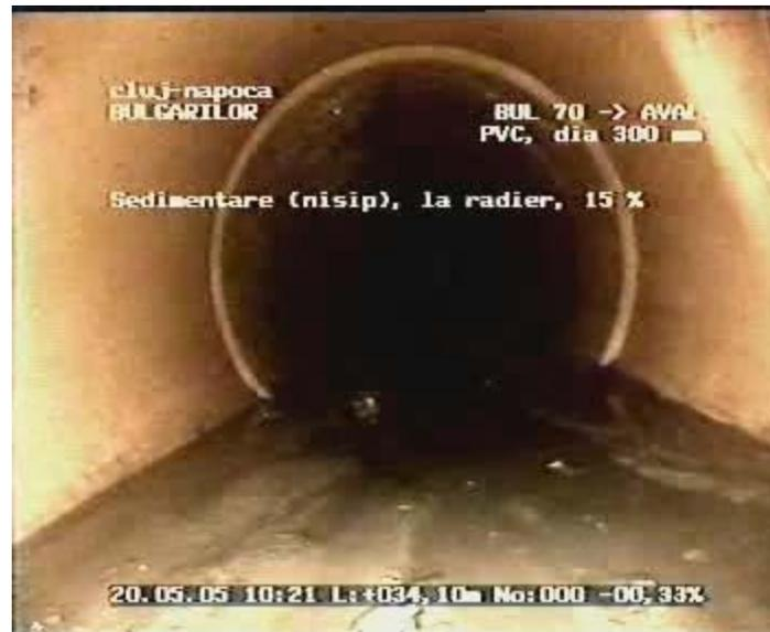
Fig. 1. Sedimentation caused by insufficient slope of the sewer pipe [2]
