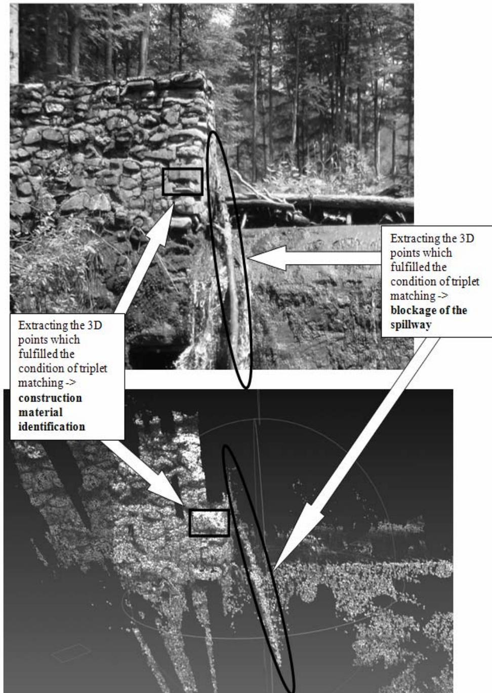
Fig. 3. *3D reconstruction of some characteristics of the dam based on 3 images stereo-restitution*
